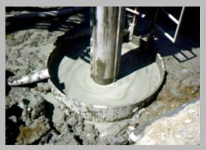
granular soils and a polymer slurry offers more advantages in cohesive soils such as clays or silts. Heavy molecular weight anionic polymers are flocculants and cannot be combined with clay which limits their use to low permeability soils.
