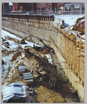
temporary supports of excavation or integrated into the design final condition at a fraction of the cost of concrete slurry walls.
