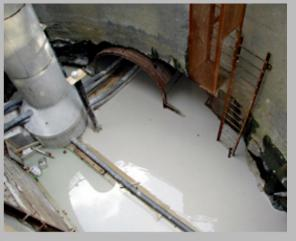
drilling and blasting, has enormous advantages over conventional methods. IMPERMIX® fills this role perfectly as a slow setting, non-shrink grout, low heat, light weight grout. The very low permeability and chemical resistance are the best protection for any buried service. Thousands of feet of tunnels have been backfilled with IMPERMIX® in 2003 in Atlanta for the new municipal drainage system.
